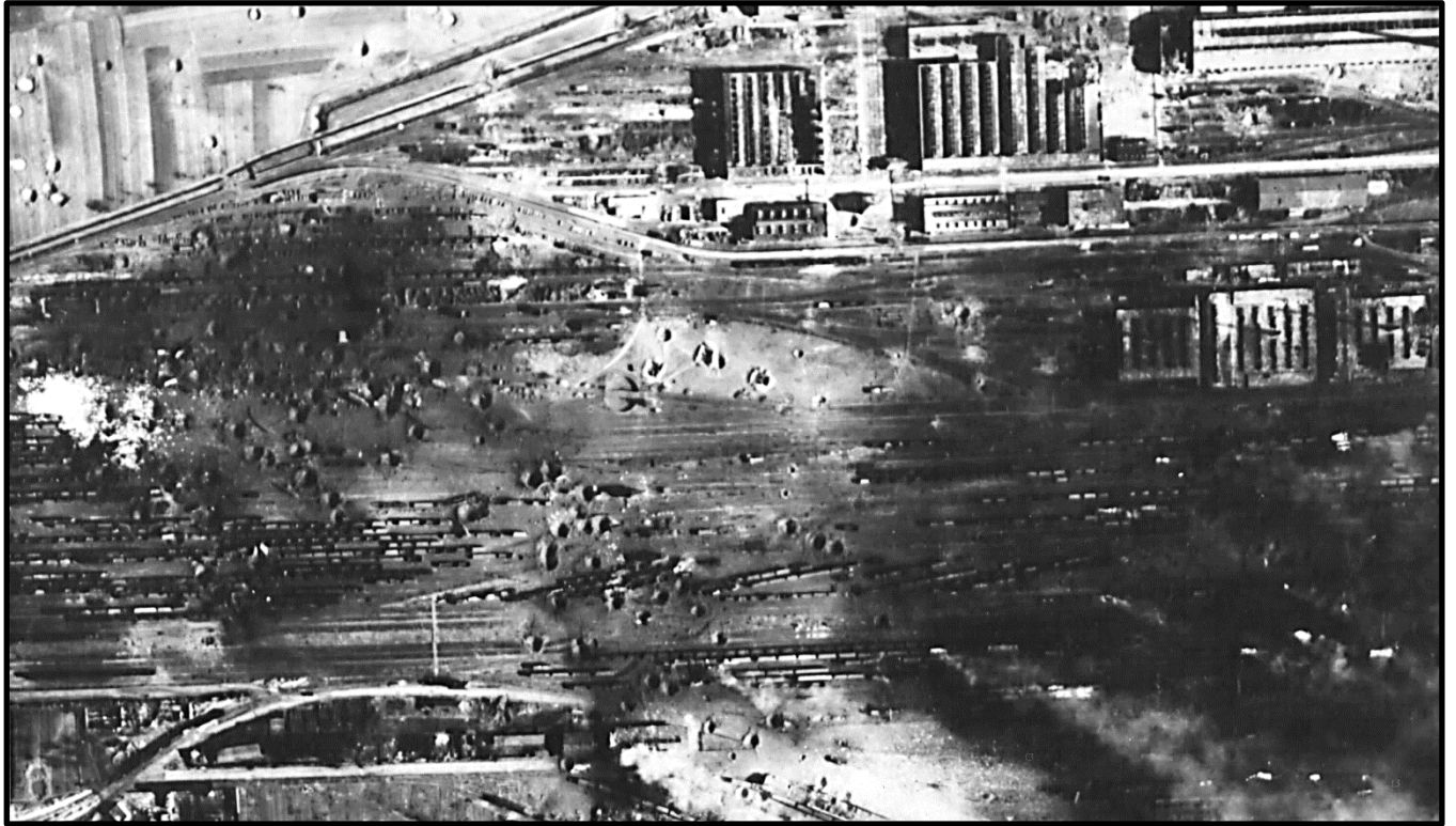
Offenburg Railroad Marshalling Yards Image courtesy of the National Archives and Records Administration ©
