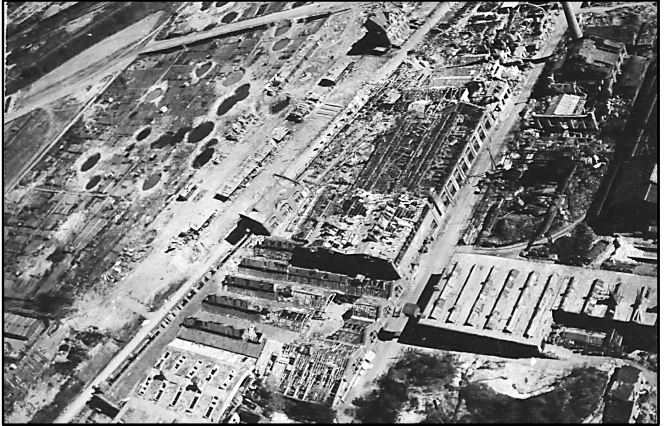
Homburg Railroad Marshalling Yards Image courtesy of the National Archives and Records Administration ©
