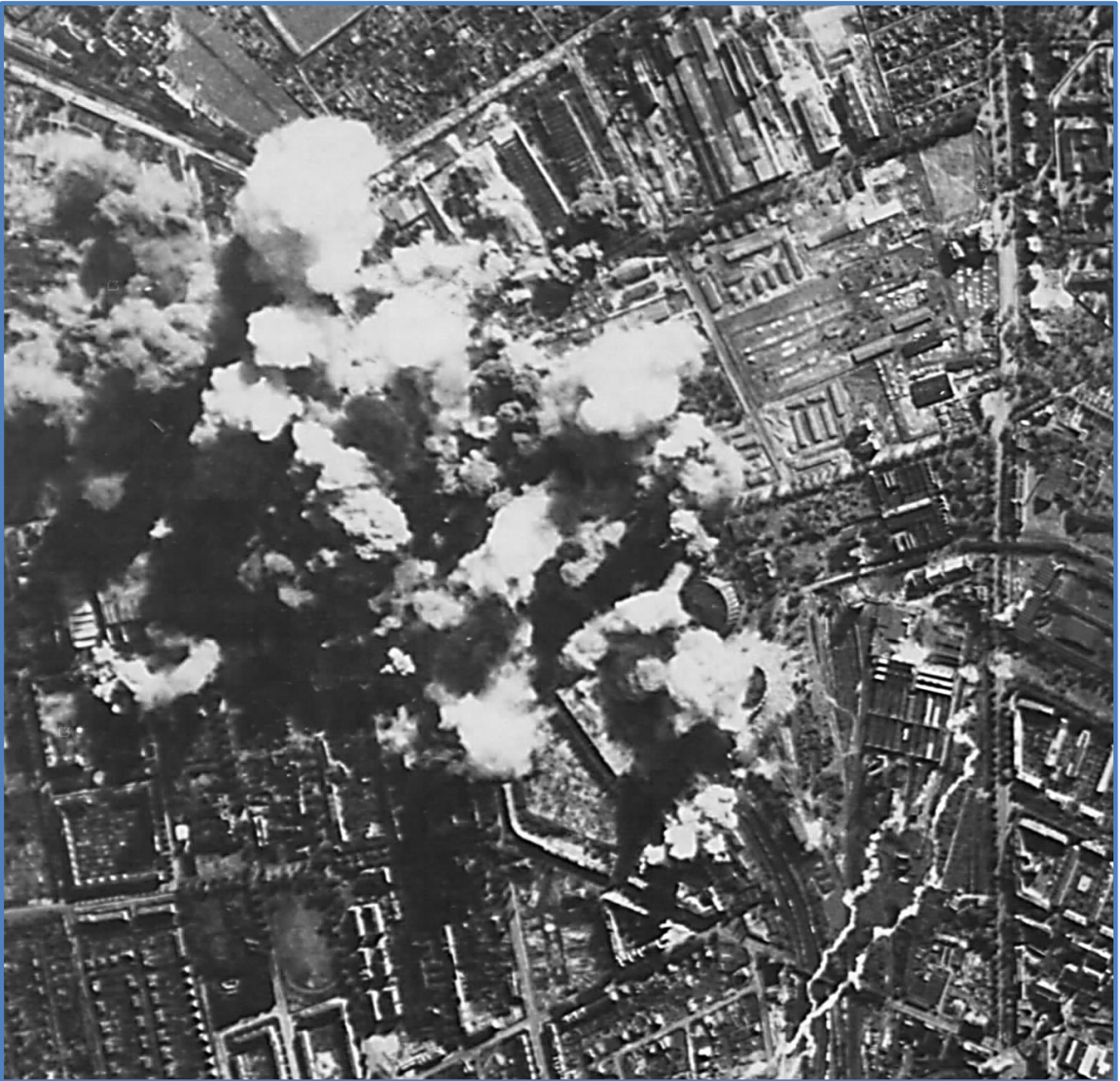
Henningsdorf Tank Factory Image courtesy of the National Archives and Records Administration ©
