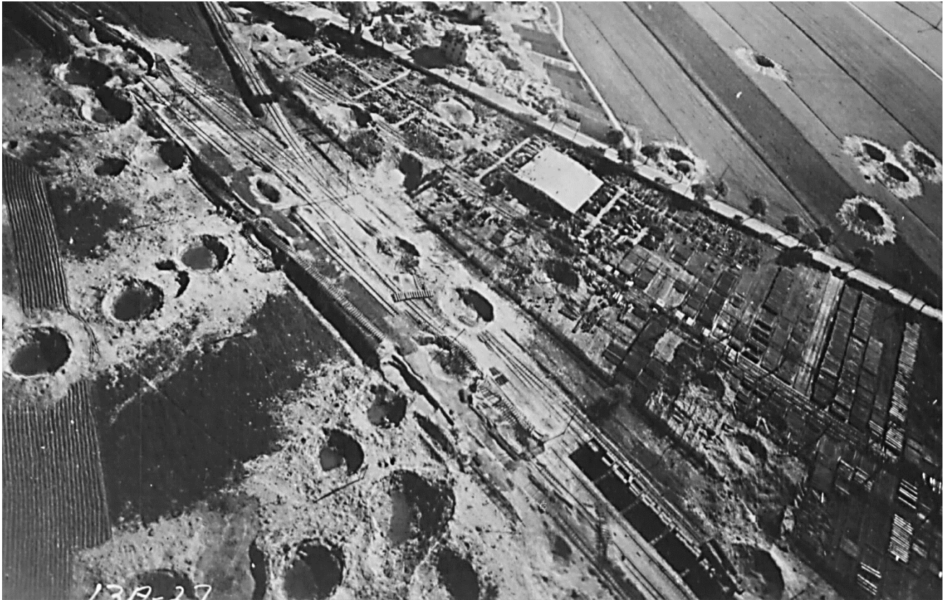
Amberg Railroad Marshalling Yard Image courtesy of the National Archives and Records Administration ©
