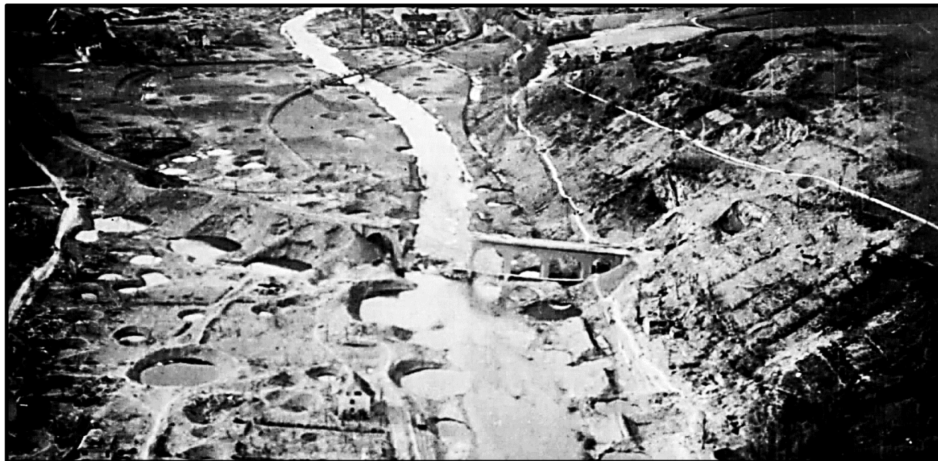
Arnsberg Railroad Viaduct is destroyed
